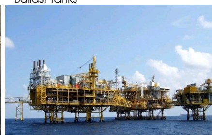
Topside and Decks
